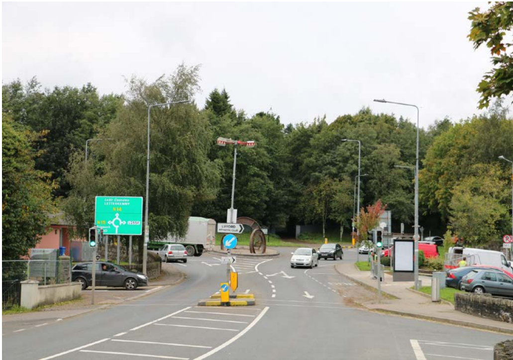
Current view – N15 in Lifford, near the Three Coins Roundabout
